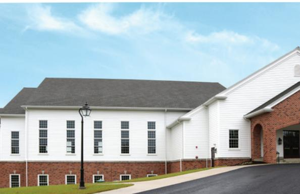
Chelsea Building Products, manufacturer of Everlast®, provided approximately 100 squares of siding in Polar White, 6-7/8" planks. The crisp white allows the red brick facade on the lower half of the building to stand out, as well as providing a stark contrast to the dark gray roof. Polar White maintains its own vibrancy too – holding its color year after year.
