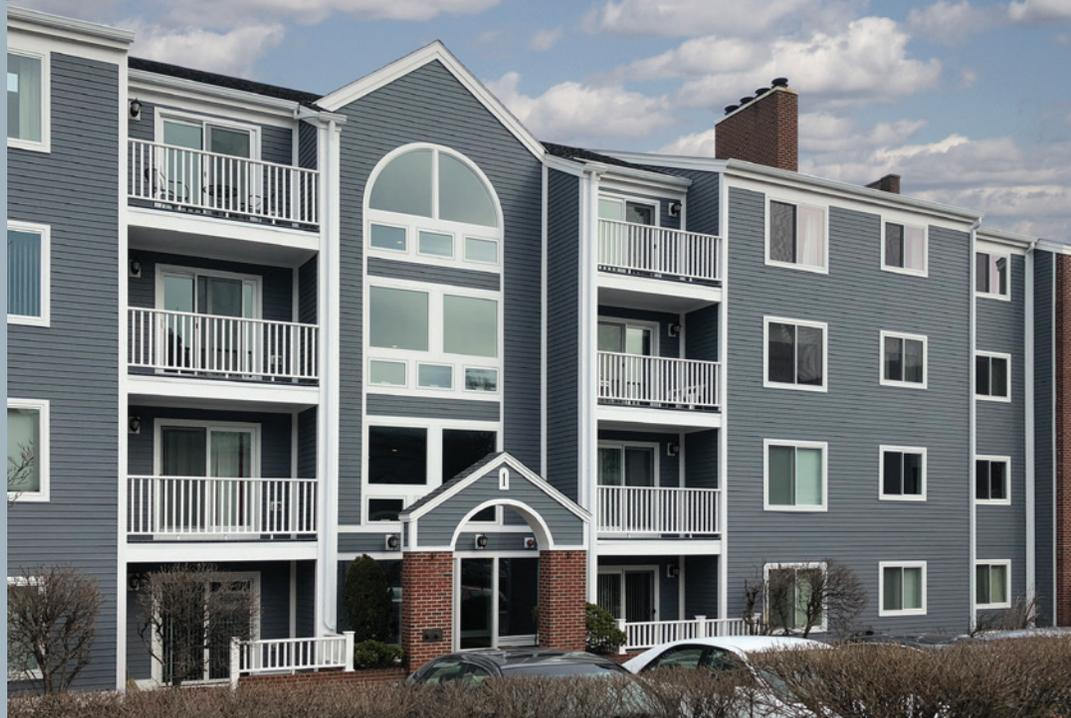
Originally built in 1980, the condominium building located at 1 Washington Street in Salem, MA recently underwent a complete building envelope replacement featuring Everlast® Advanced Composite Siding, 4-½ inch planks in Flagstone color.
