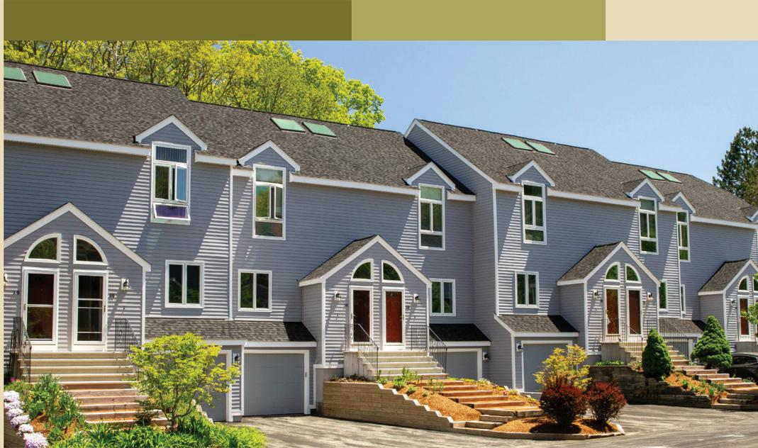
Hager Meadows is a 10-building, 84-unit condominium complex located in Marlborough, MA. The homes were built in 1988 with an exterior that was constructed of low-grade cedar siding, a material that breaks down after yearly freeze-thaw cycles in climates such as the one in Massachusetts.
