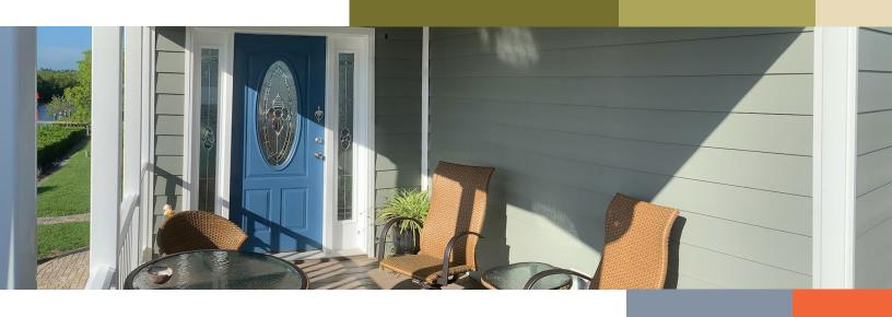
Because the home is located within a hurricane zone, a key selling point was Everlast siding's wind resistance. The product is rated to withstand winds of up to 198 miles per hour when installed with screws and 175 miles per hour when fastened with nails.
