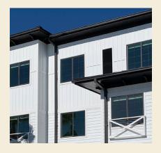
Everlast® Siding: 7" lap siding and Everlast Board & Batten
